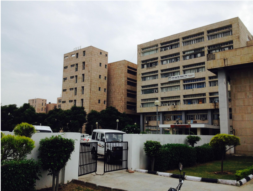
Figure 3 The Department complex is a set of two interconnected 6 storey buildings
